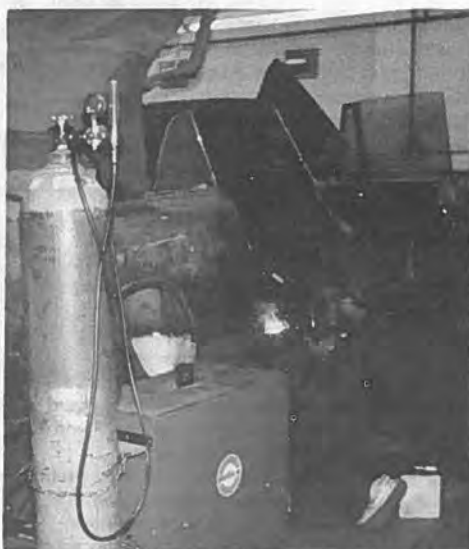
Stripped bare and now panels hand made and welded in place.
