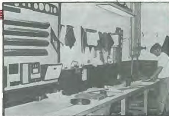
A corner of the woodwork shop. The operative is making up a picnic table for the rear seat of a Silver Spur. Note the specimen panels on the wall.
